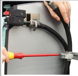
Fix the second core of the DC link connecting cable to the profile rail using a cable clamp.
