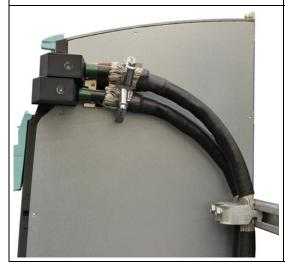
The installed DC link connecting cable is shown in the adjacent diagram.
