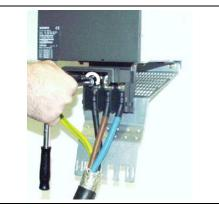
Attach the protective conductor and the power cable.
