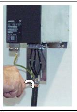
Tighten the hose clamp at the shield connecting plate.
