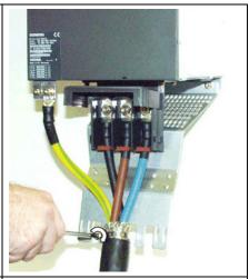
Tighten the hose clamp at the shield connecting plate.
