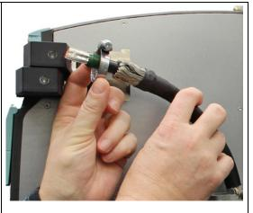
1. Fix the first core of the DC link connecting cable to the profile rail using a cable clamp.
