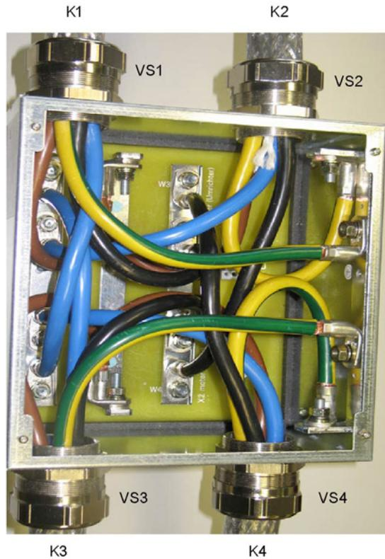
Figure 10-17 Wired Voltage Protection Module VPM200 Dynamic with short designations
